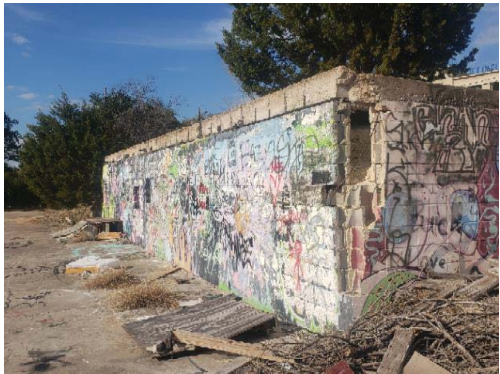
Figure 04. Blowout at corner in upper wall
