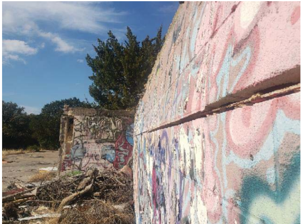
Figure 03. Faulting of upper wall
