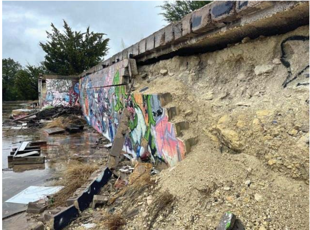
Figure 02. Partial collapse and buckling of upper wall
